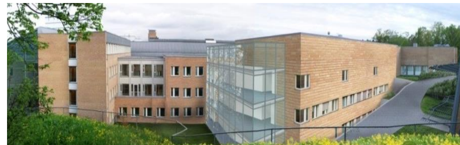
Manufacturing facility at Gaustad
