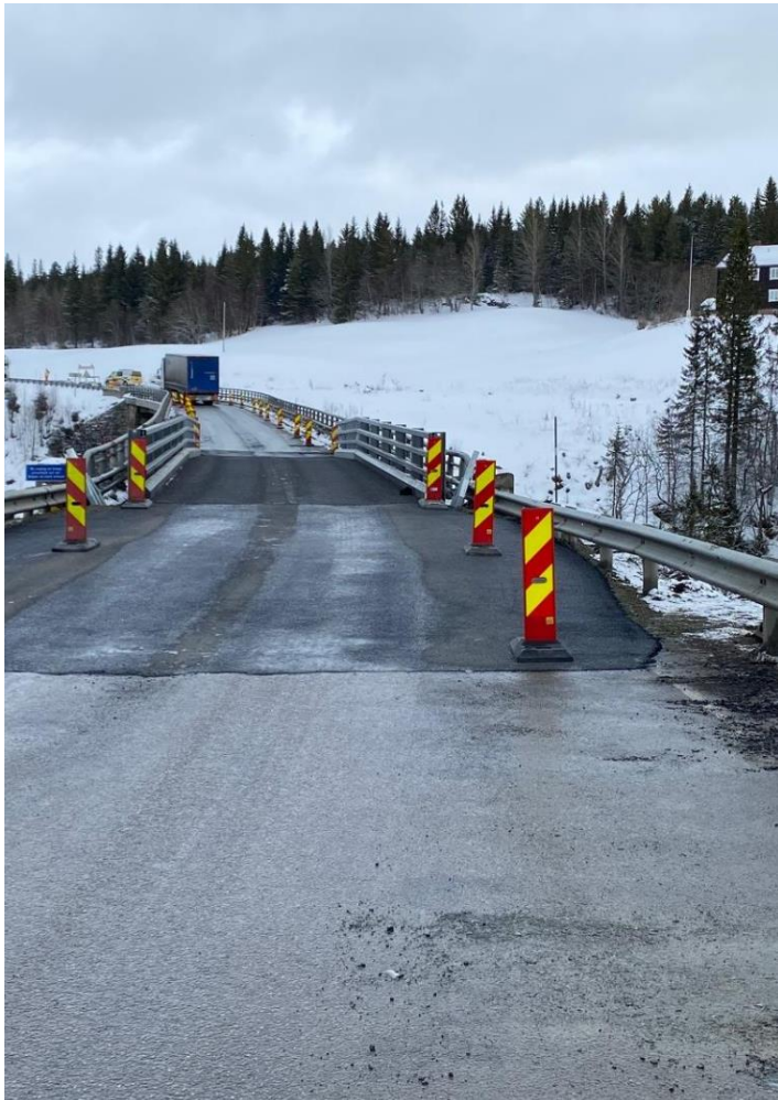
14/4-21: Interrim bridge in place
