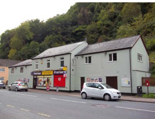
External view of "Central Stores"
