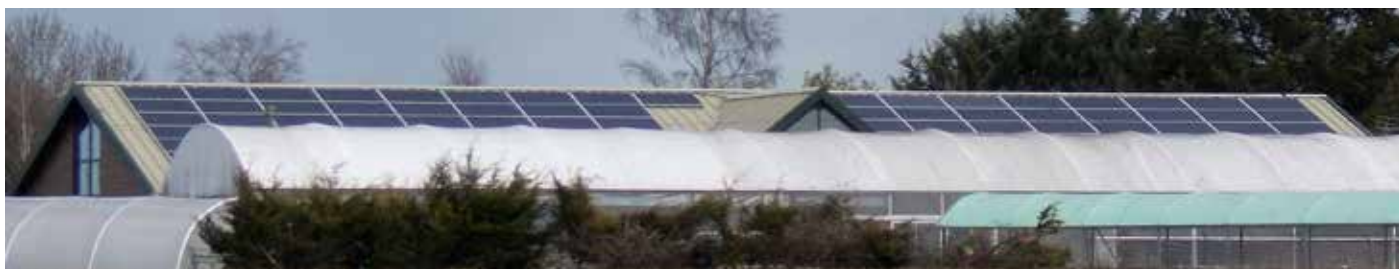
Staunton Garden Centre PV
