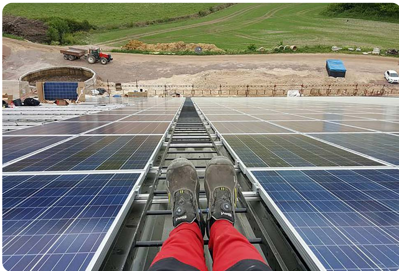
Nöbble Gård solar farm. Photo Kalmar Energi.
