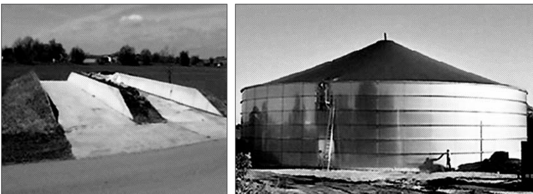
Figure: Storage space (silo) for energy crops and manure storage (covered) (Photo: Kaiser Baustoffwerke, Sammer Werksvertretung)
