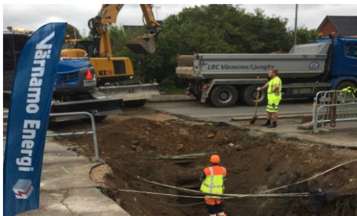
Figure 6 Digging under the main road in Bor, for the new grid. Photo: Värnamo Energi.
