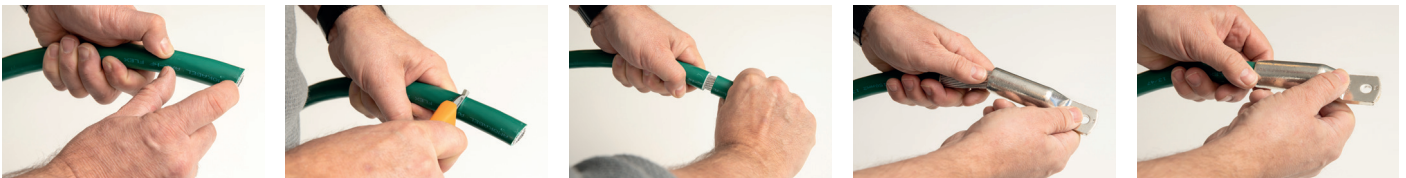
Stripping of insulation.
