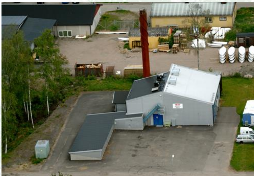
Figure 12 - District heating plant in Rottne
