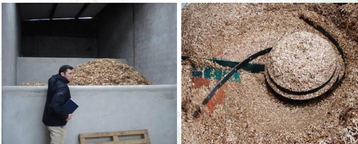
Figure 50 - Fuel store and agitator at Gurteen Agricultural College
