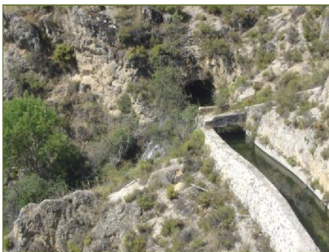
Figure 45: Channel-tunnel. Central Potril II. Granada
