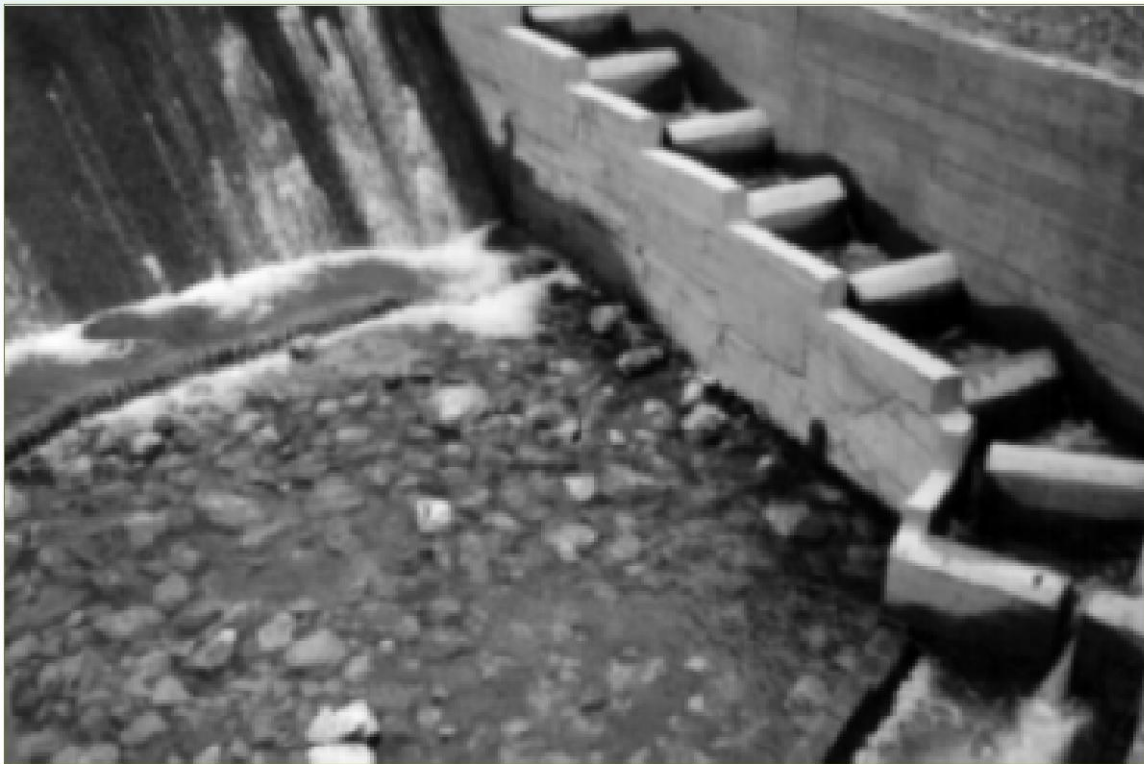
Figure 52: Fishpass with vertical slots (Source: ESHA)
