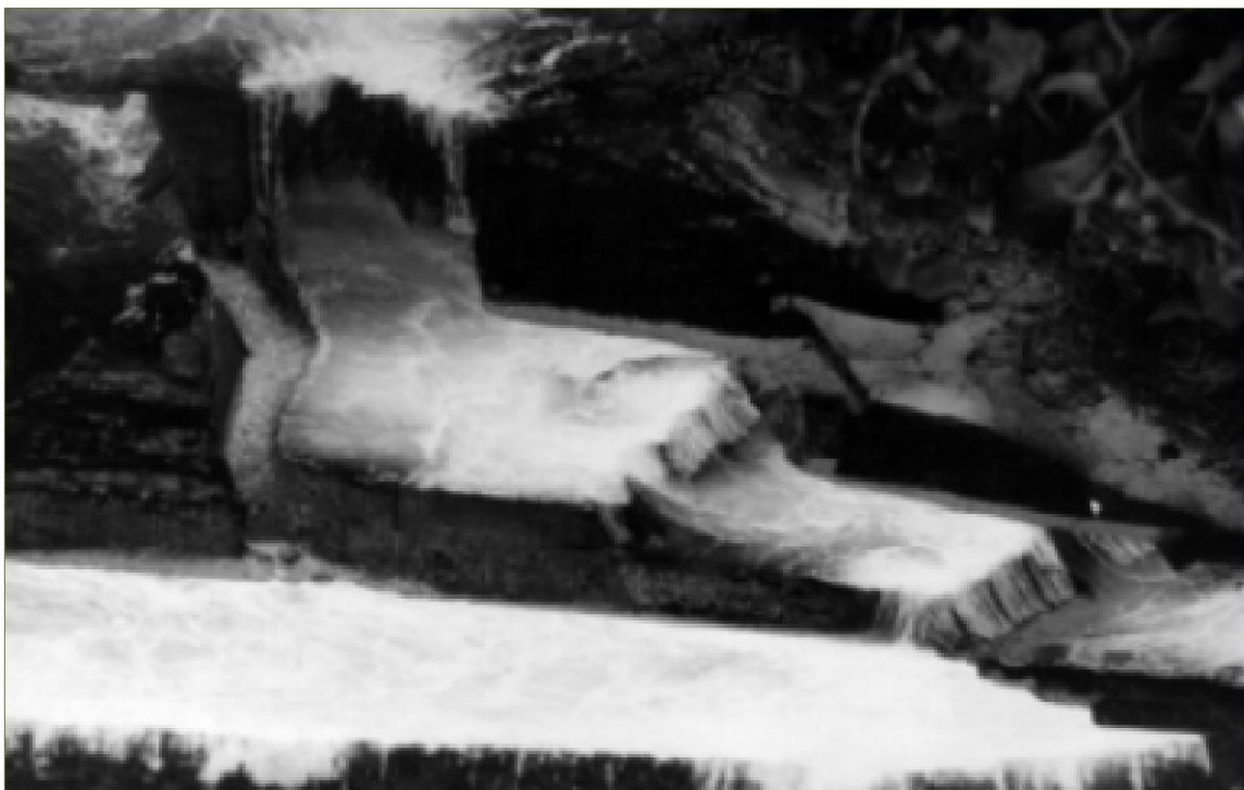
Figure 52: Fishpass with vertical slots (Source: ESHA)
