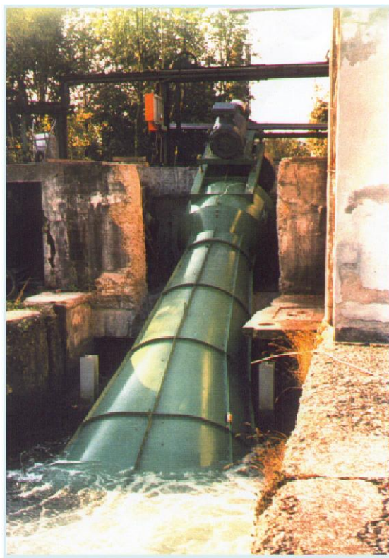
Picture 14: Suction Tube (Source: Saltos del Pirineo SL)
