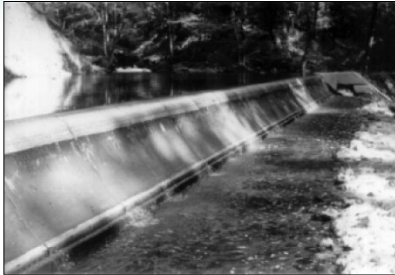
Figure 60: Self-cleaning screen (Source: ESHA)
