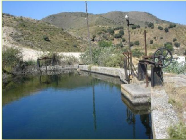
Figure 46: Forebay. Central Potril II. Granada
