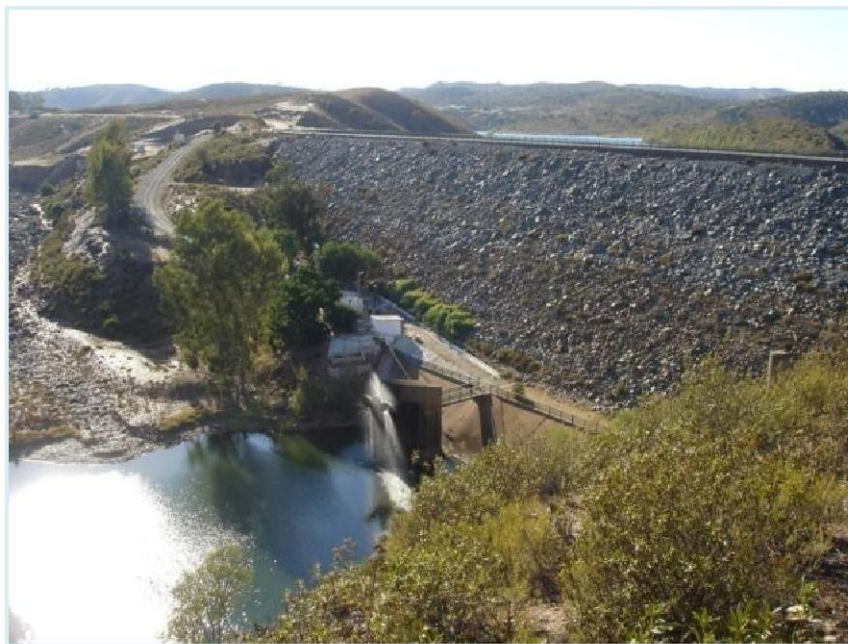
Picture 8: Earth dam. Agrio Dam. Seville.
